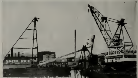
Smith-Rice Derrick Barges Nos. 3 and 4, raising a third derrick barge which recently sank in Islais Creek. The sunken derrick barge is owned by a local construction company. The lift was 178 tons.
